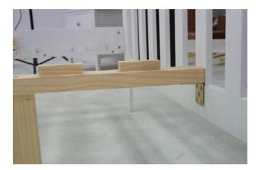
13. On the other end of the centre support rail align the end of the rail with the foot board of the bed.
