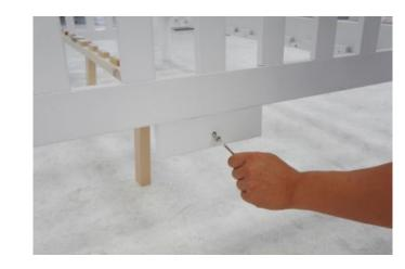
12. After ensuring all the grooves align. Connect the top end of the centre support rail with the panel beneath the bead head, fit the small metal bolt through the hole and tighten.
