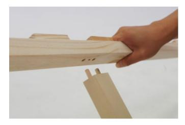
9. Gather the centre support rail and support legs, insert 2 thinner wooden dowels to the timber legs and connect them to the bottom of the centre support rail.
