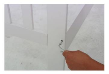
5. Use the Alan Key provided in the hardware pack to firmly tighten the metal bolts, please ensure you do not over tighten
