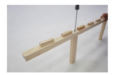
INSERT a screw through the hole positioned at the top of the centre support rail, TURN & FULLY TIGHTEN with screwdriver to secure the legs below (Important). Repeat for all 3 legs.
